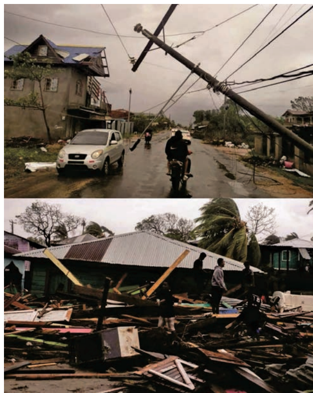
Fig. 9 Hurricane Iota and its passage through Nicaragua: Hurricane Iota's winds affected the infrastructure (upper photo) and housing (lower image) in Puerto Cabezas. Source: BBC News.
