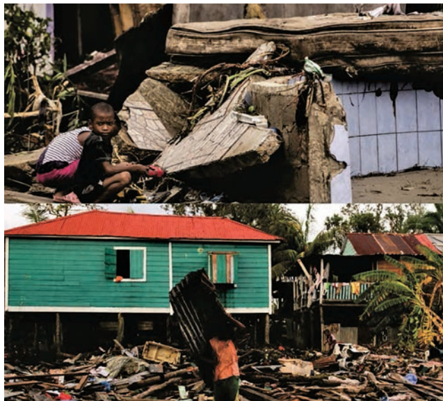
Fig. 8 Effects of Hurricane Eta in Nicaragua: Children in Puerto Cabezas after Hurricane Eta (upper photo). Source: UNICEF); Debris of destroyed houses after the passage of Eta (lower image). Source: ONU News.
